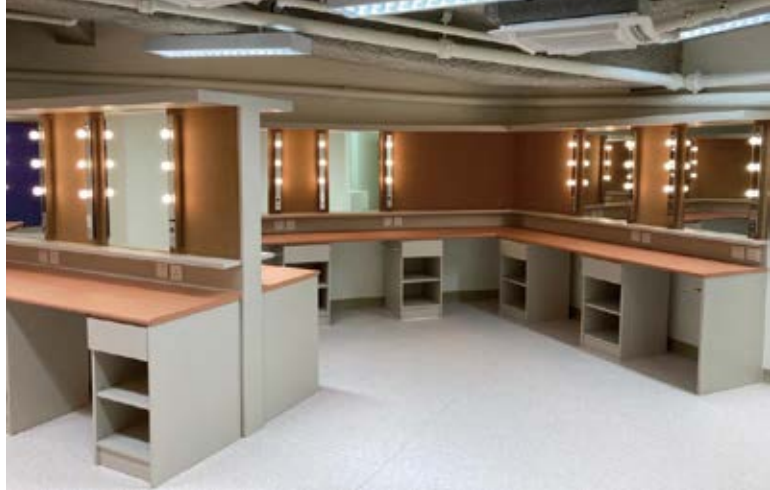
Renovation of four dressing rooms has been completed in August 2020. 四個化妝間在 2020 年 8 月完成裝修。
